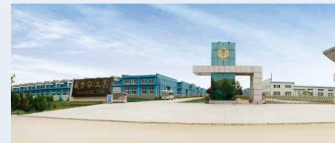
威海临港新区厂区 Weihai Lingang New District Factory
